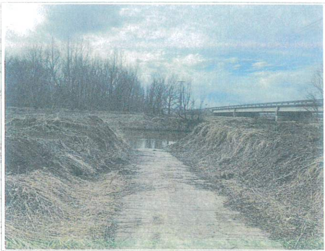
Looking South down boat ramp, trees have been removed.
