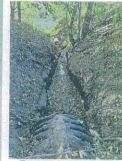
3 EXISTING STORM PIPE LOOKING SOUTH
