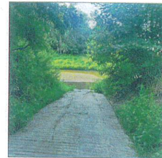
1 EXISTING BOAT RAMP LOOKING SOUTH
