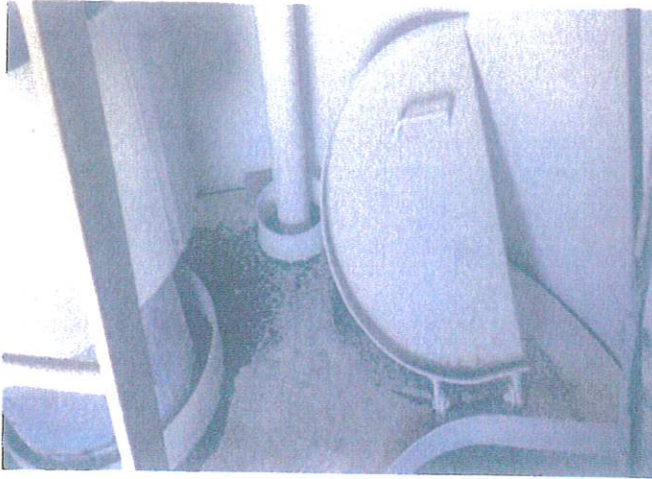
Dry Interior Coating
