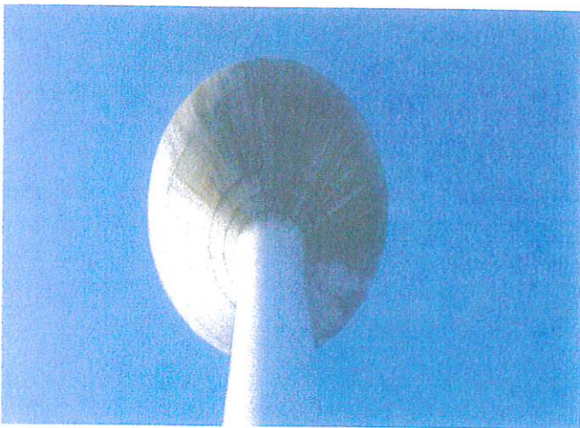
Exterior Under Belly and Pedestal Coating
