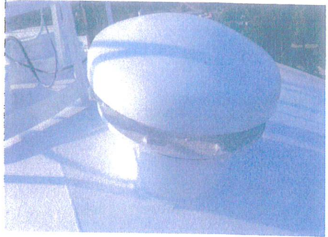
Roof Vent Structure
