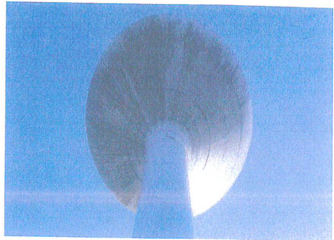
Exterior Under Belly and Pedestal Coating
