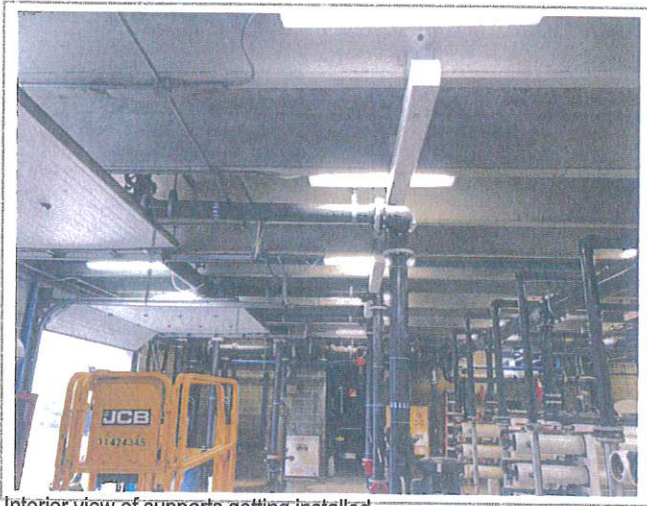
Interior view of supports getting installed
