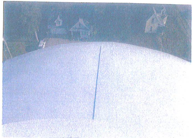
Exterior Roof Coating
