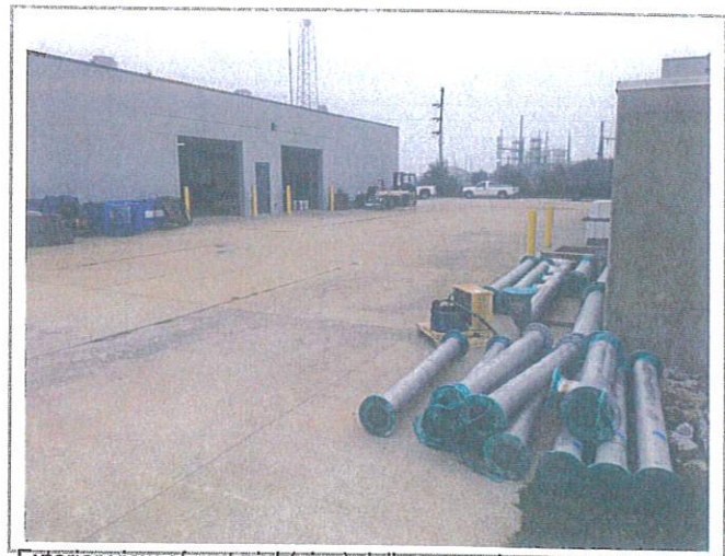
Exterior view of material (pipe) delivery on site
