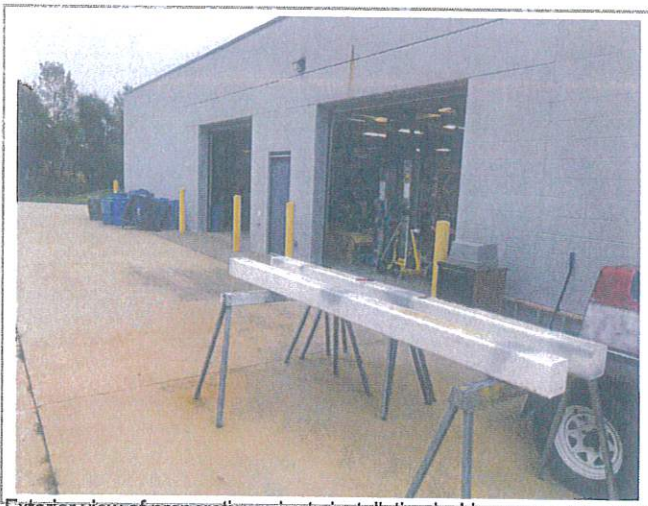
Exterior view of preparation prior to installation inside
