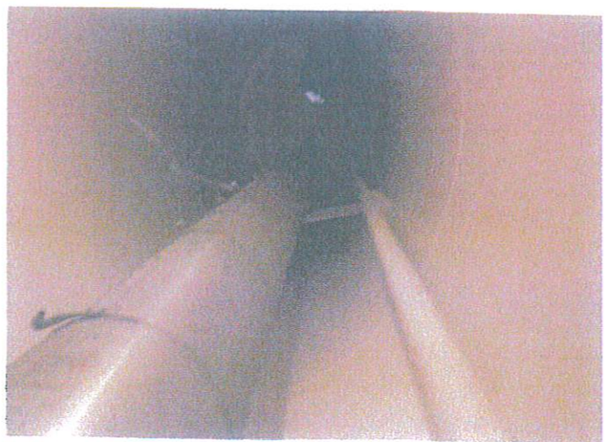
Dry Interior Coating
