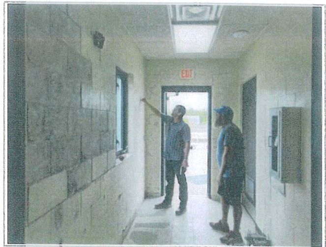
Overview of the entrance - grinding has progressed into this space
