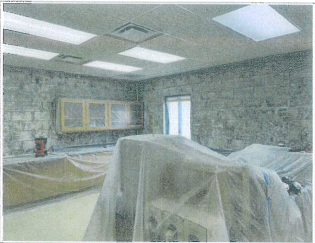
Overview in the lab shows wall grinding is nearly complete
