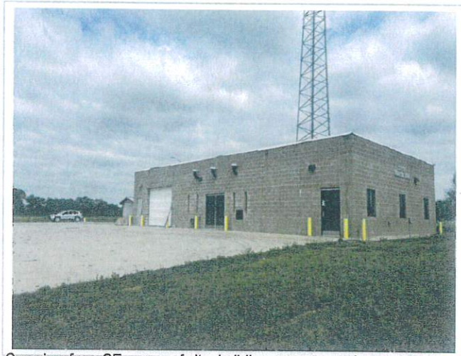
Overview from SE corner of site, building appears unchanged from last visit
