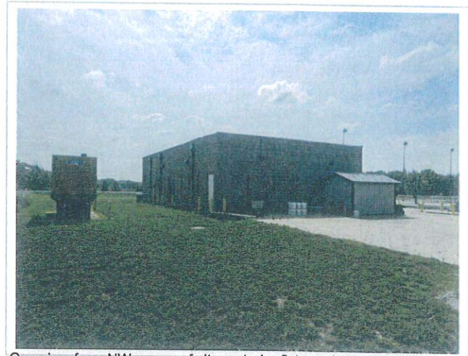
Overview from NW corner of site, exterior fixtures have not been removed or prepped for upcoming work
