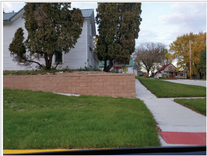
Example of retaining wall within private property without railing in Riverside.
