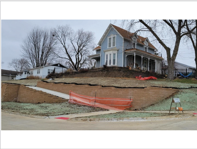
Requesting that some type of safety rail or fence be placed on top of the retaining wall within the private property.
