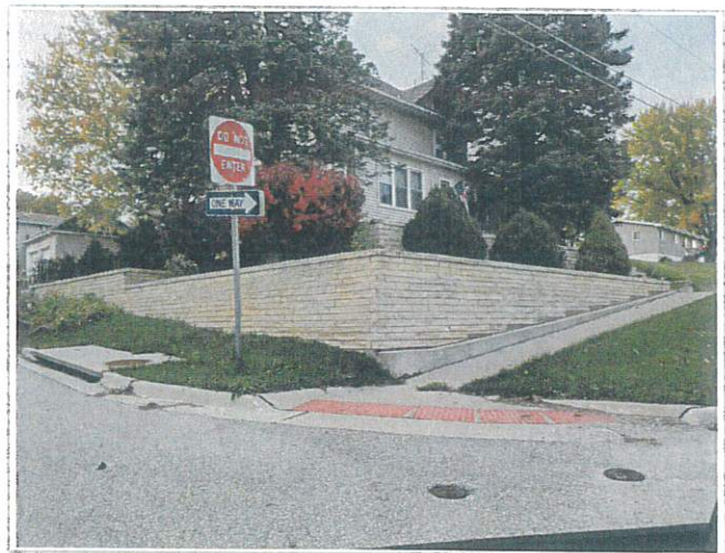
Example of retaining wall within private property without railing in Riverside.
