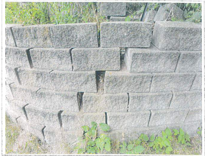
Zoomed in view of existing retaining wall condition prior to construction.
