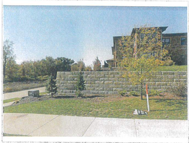
Example of retaining wall within private property without railing in Iowa City.
