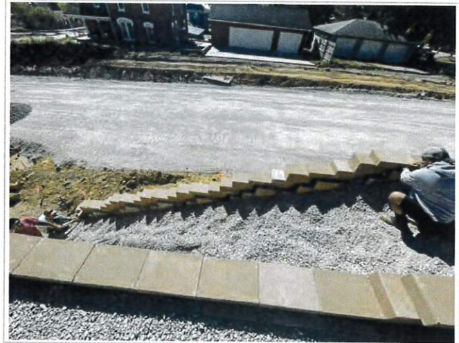
Kevin's Concrete pulling string line for the stairs located in the retaining wall
