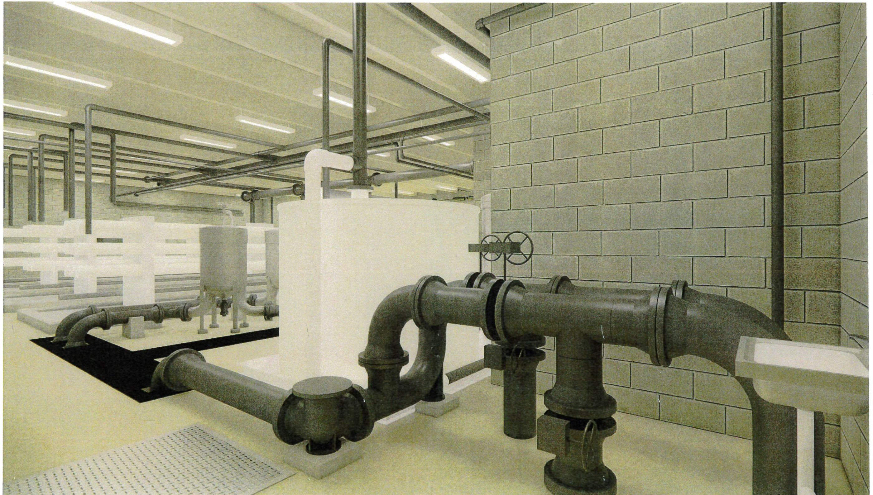
Raw Water Supply Piping Riverside WTP Pipe Improvements
