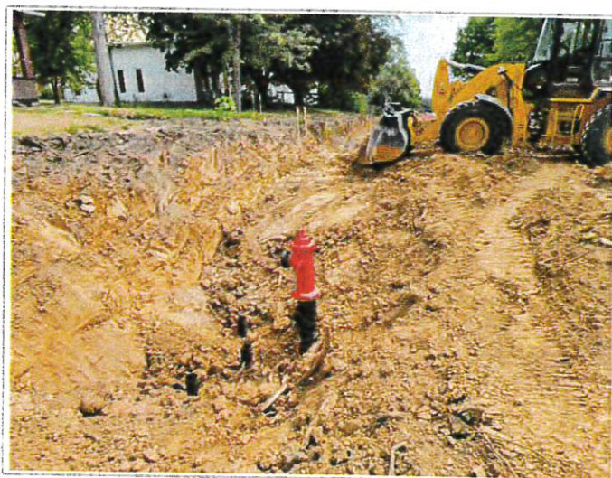
Hydrants have been installed at NE corners of Washburn and Glasgow
