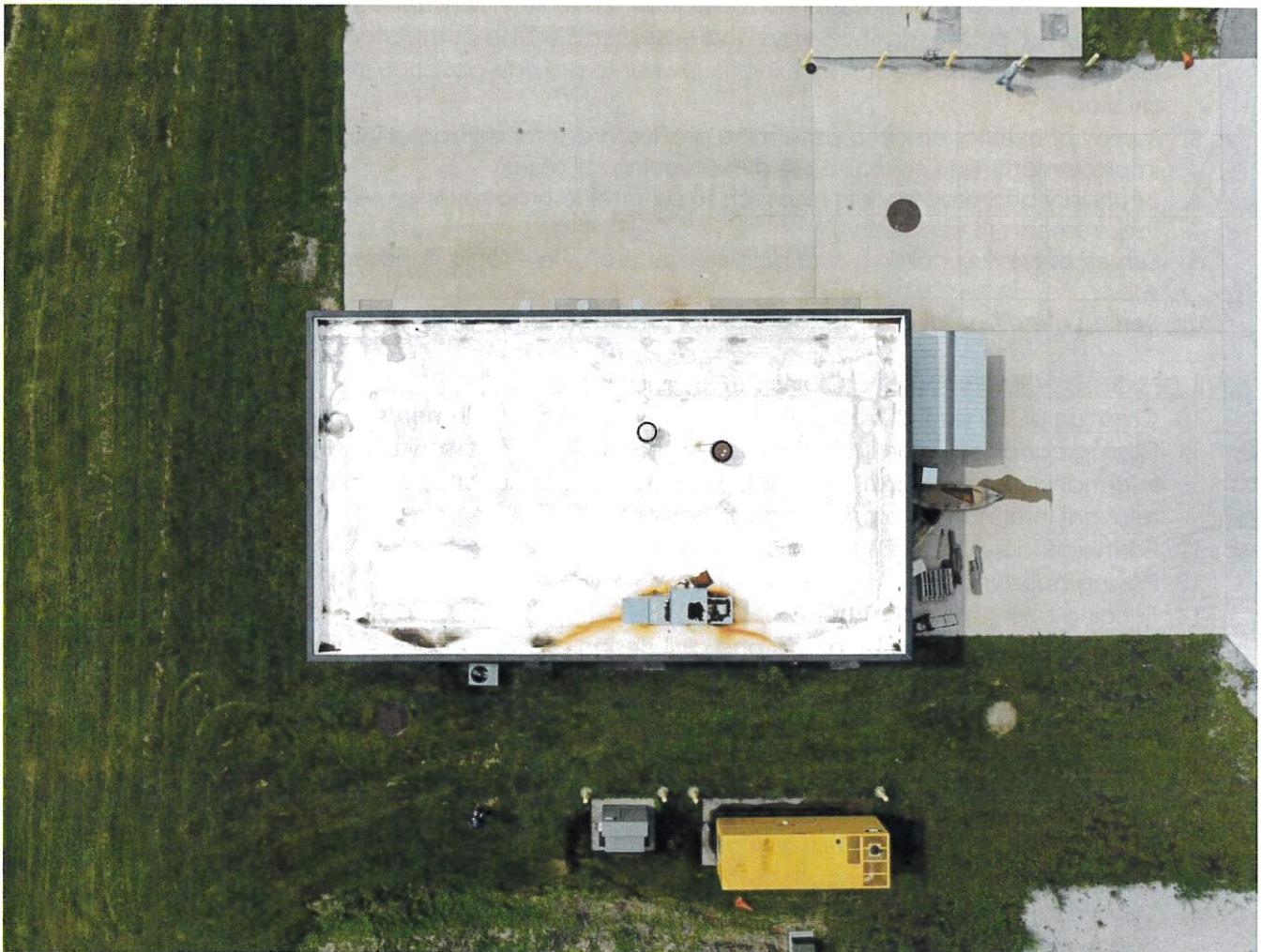
image of WWTP during PCA investigation
