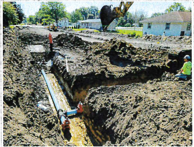
Carter Associates installing water mains and hydrants throughout Phase 1
