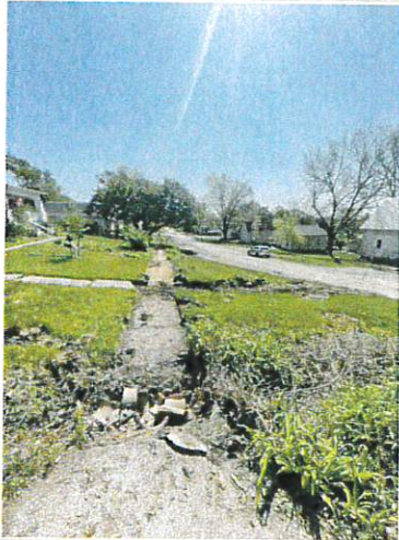
3rd & Greene, looking east down north sidewalk removals along 3rd
