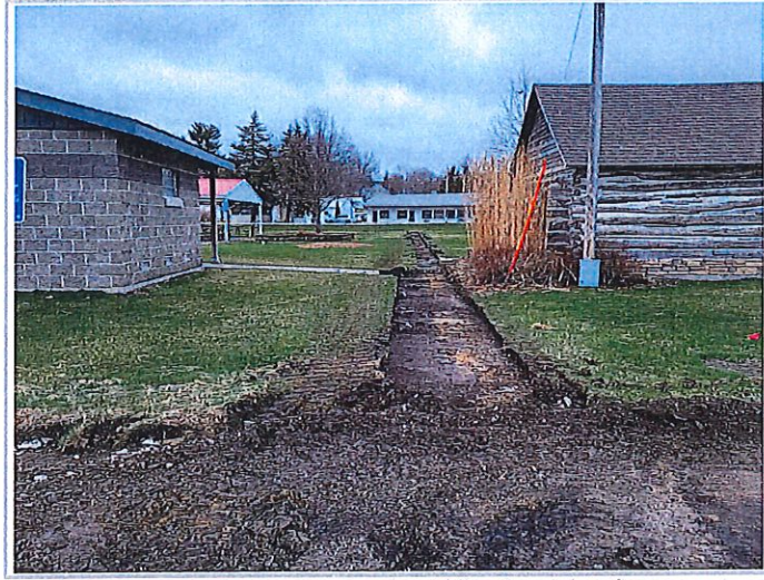
Looking north, concrete path through middle of park has been removed
