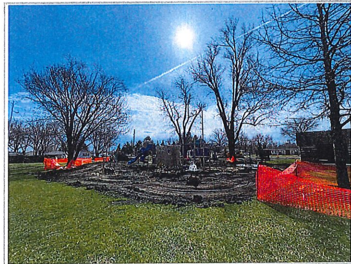
Playground area with all sand removed.
