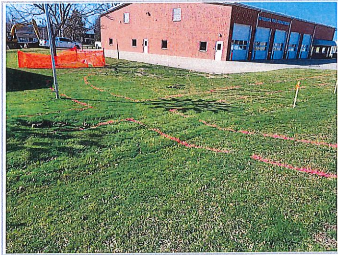
Sidewalks marked out in the NW corner of the park
