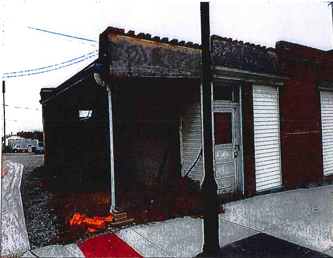
1st Street Garage
